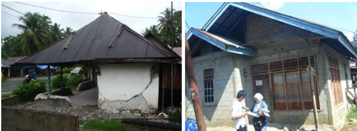
Figure 21 (left). Example of unreinforced masonry construction from Padang. In this case the house was built from river stone and mortar with no reinforcement.
